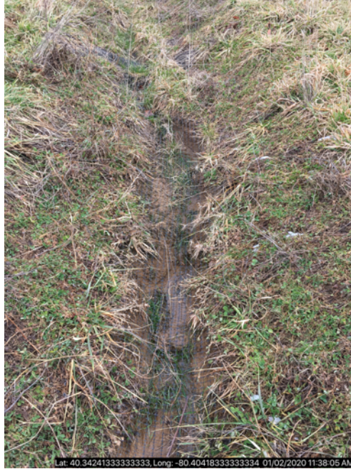
Photo #3 Accelerated erosion channel in interceptor channel 2
