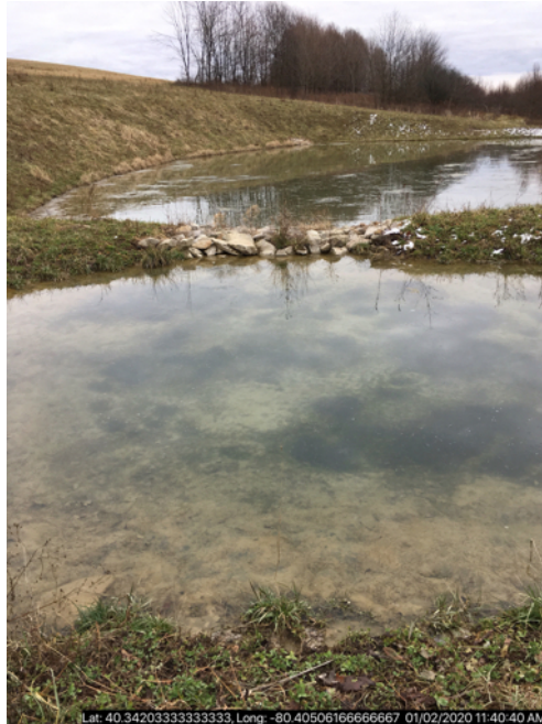
Photo #3 Accelerated erosion channel in interceptor channel 2
