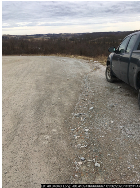
Photo #2 Accelerated erosion channel at access road entrance
