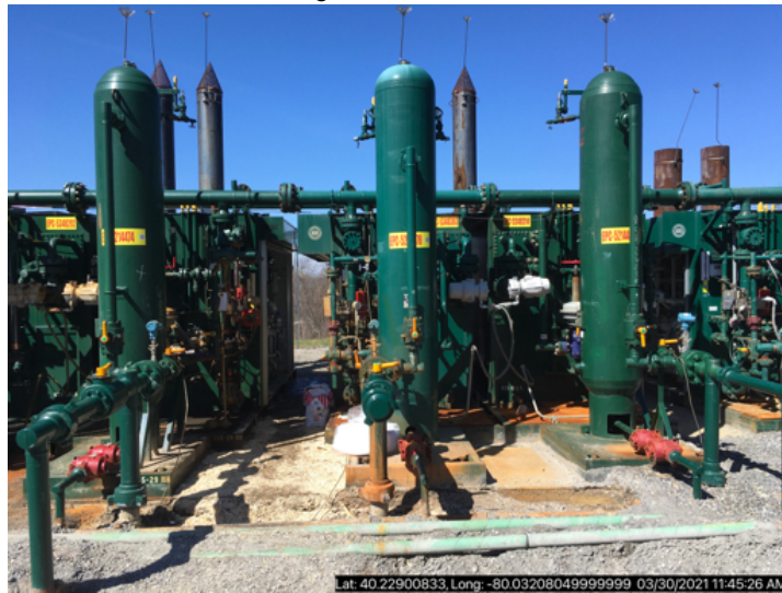
Photo # 6: previous remediation in front of GPUs
